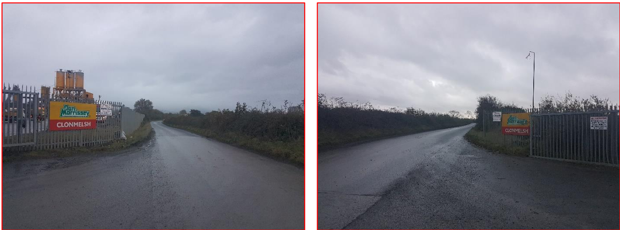
FIGURE 2-1: L3050 TO THE WEST (LEFT) AND EAST (RIGHT) AT SITE ACCESS
